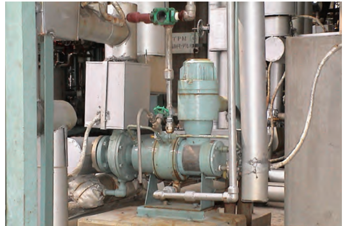
High-temperature type pump in a chemical plant.
