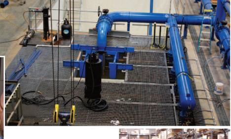
With horsepower ranges up to 500 HP and capacities to 35,000 GPM, EFH's cast iron submersible pumps meet a wide range of industrial, municipal, flood control, and residential water and wastewater applications. The cast iron line of pumps includes submersible sewage, submersible sump, semi-vortex, vortex, grinder, non-clog, and dry pit models.
